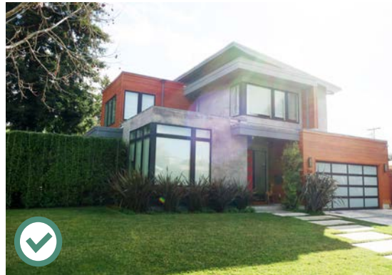
New construction with concrete and vertical wood cladding that takes cues from mid-century modern design. This home on a corner lot has windows that face out toward the street, away from neighbors.
