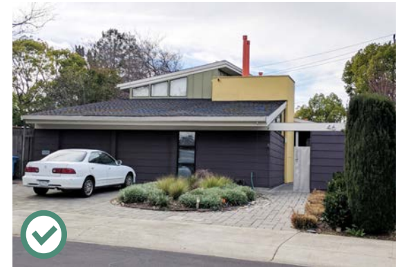
New construction with simple horizontal and vertical cladding and smooth cladding. In addition, this example uses flat and shed roof forms, and window forms that are compatible with surrounding Eichler houses.
