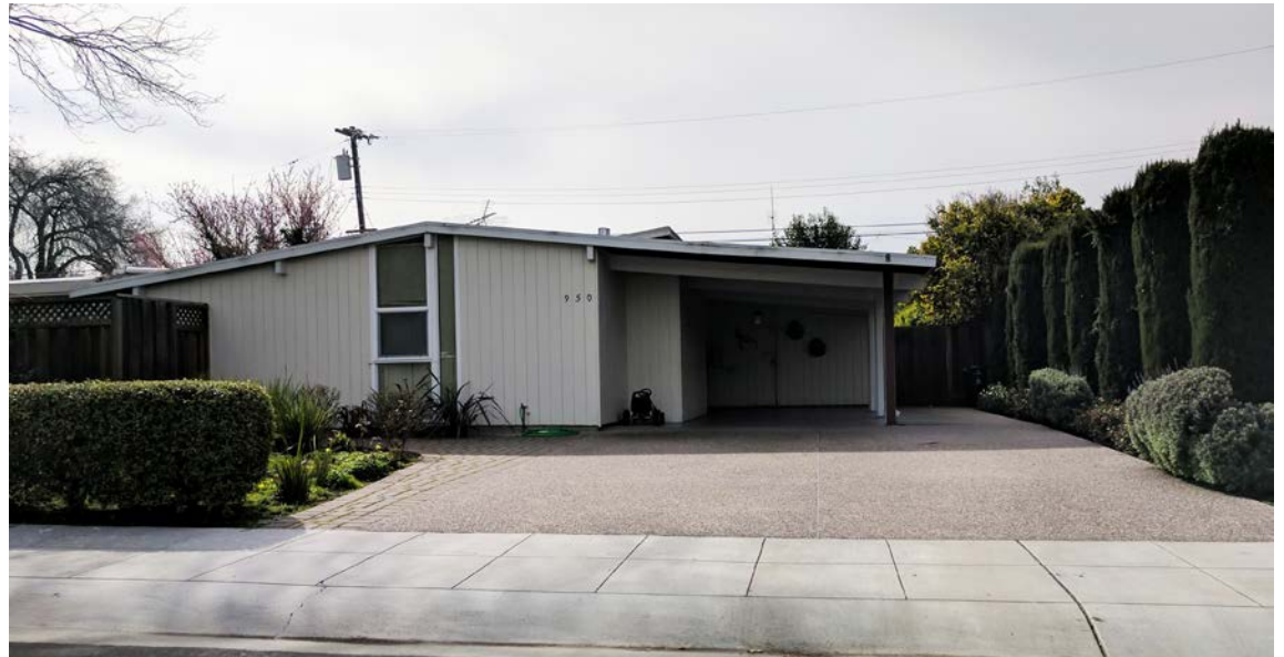
Vertical wood board siding is characteristic of Eichler houses, though the width of the boards varies.
