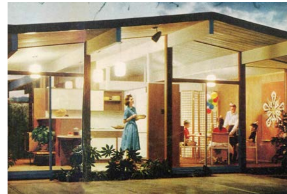
Top: A well-recognized Eichler house design features angled clerestory windows.
