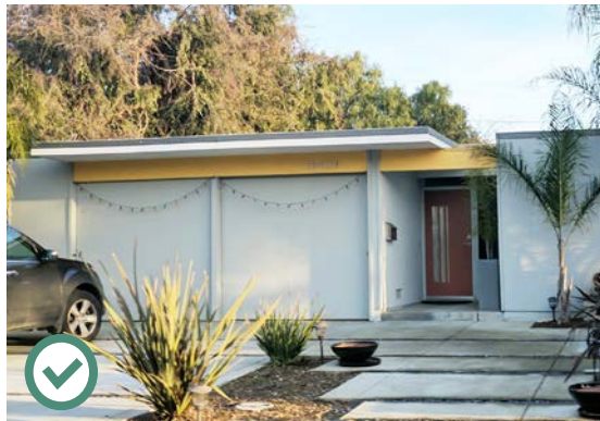
Example of vertical scored garage doors and an appropriate replacement door. The door is flush and has only minimal rectangular lites in a modern style.
