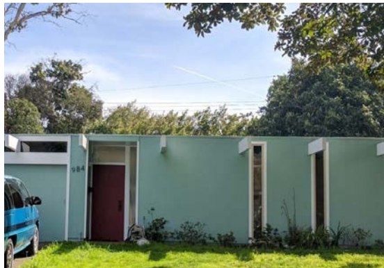
Top: Eichlers typically feature vertical board siding, and some, like this example, also use concrete block.
