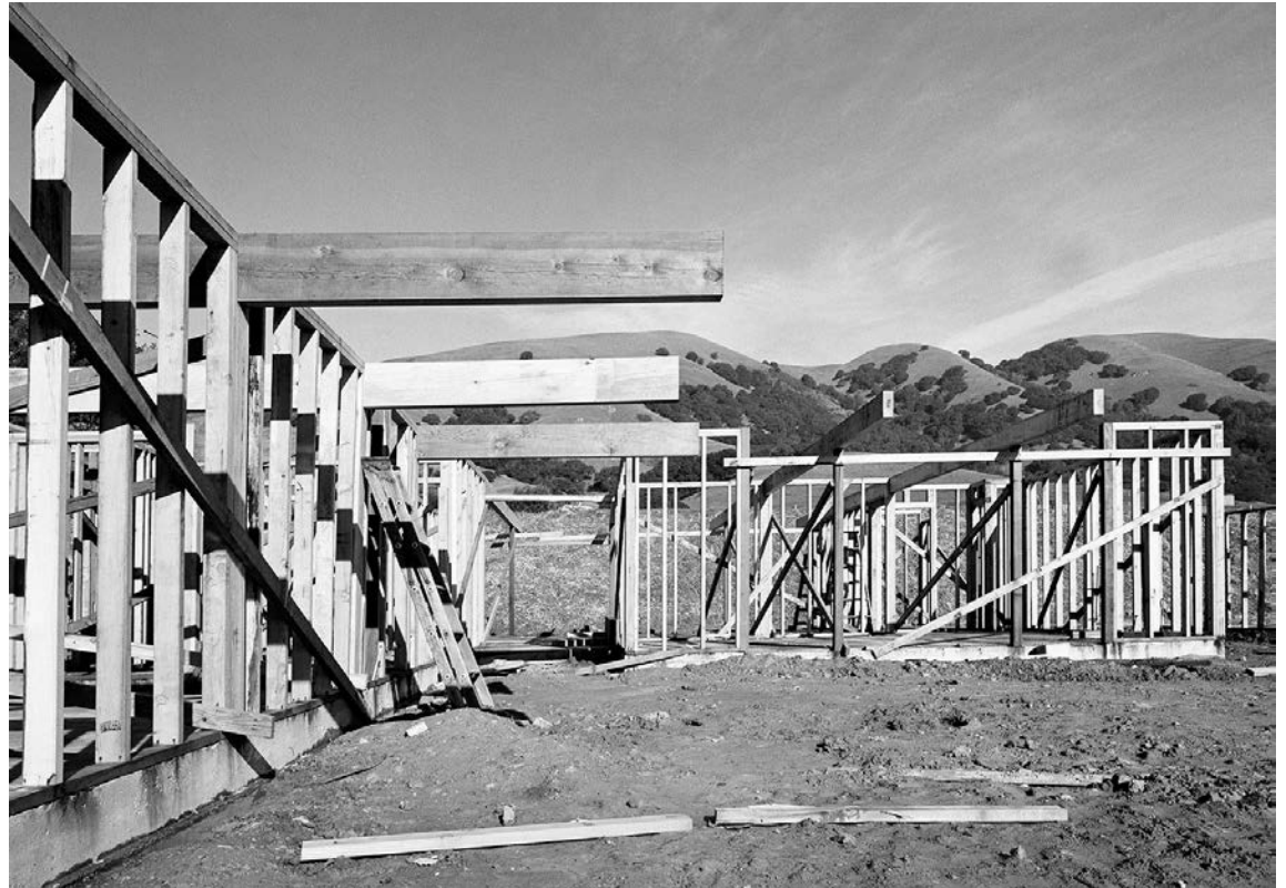
The post and beam construction method is evident in this photograph, 1950s. Credit: Photograph by Ernest Braun.
