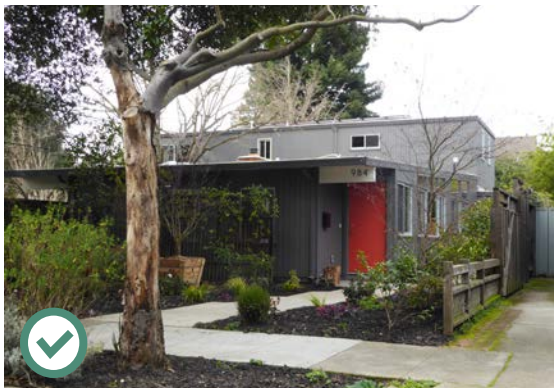
Second story addition at the rear with vertical wood siding that is similar to, but does not directly copy, the cladding of the original portion of the Eichler house.
